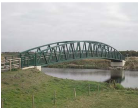
The recently constructed Four Mile Bar Bridge
