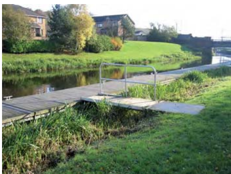
Example of 'soft edge' pontoon installation, Forth & Clyde Canal
