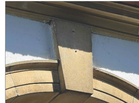
Removed fixing marks on keystones (typical)
