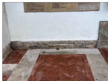
View of Brick Panel 4 from north. Crack in stone section 3 visible on left.
